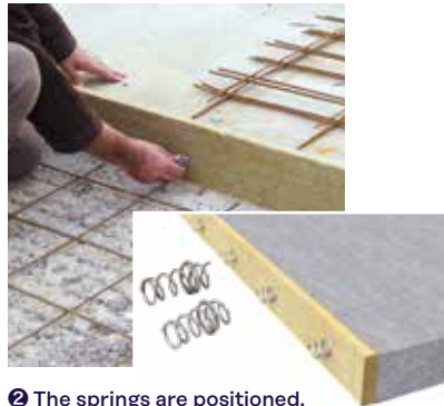
❷ The springs are positioned.
