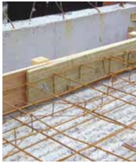
❶ The strips are nailed to the edge formwork.
