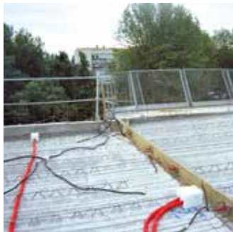
❶ Phase 1 Titan dowel positioning.
