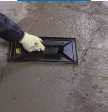
Talochage de Mapegrout SV Fiber
