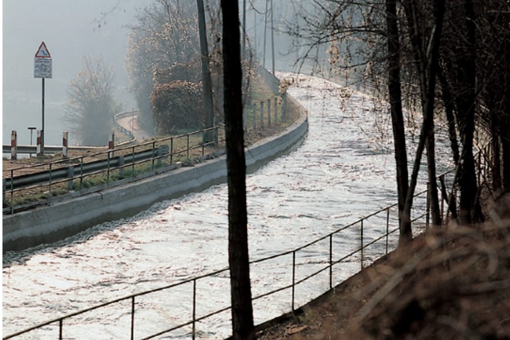
Bertini hydroelectric canal - Como - Italy. Surfaces treated with Planiseal 88
