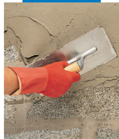
Application of Planiseal 88 by trowel
